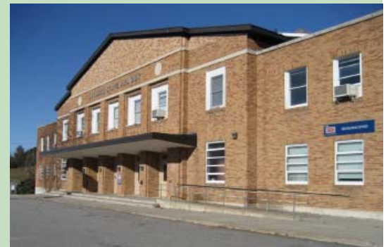
Maine Army National Guard Armory Augusta, Maine
